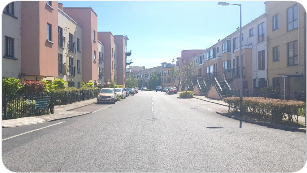
Figure 6 – Longfield Road (view to south from subject site)
