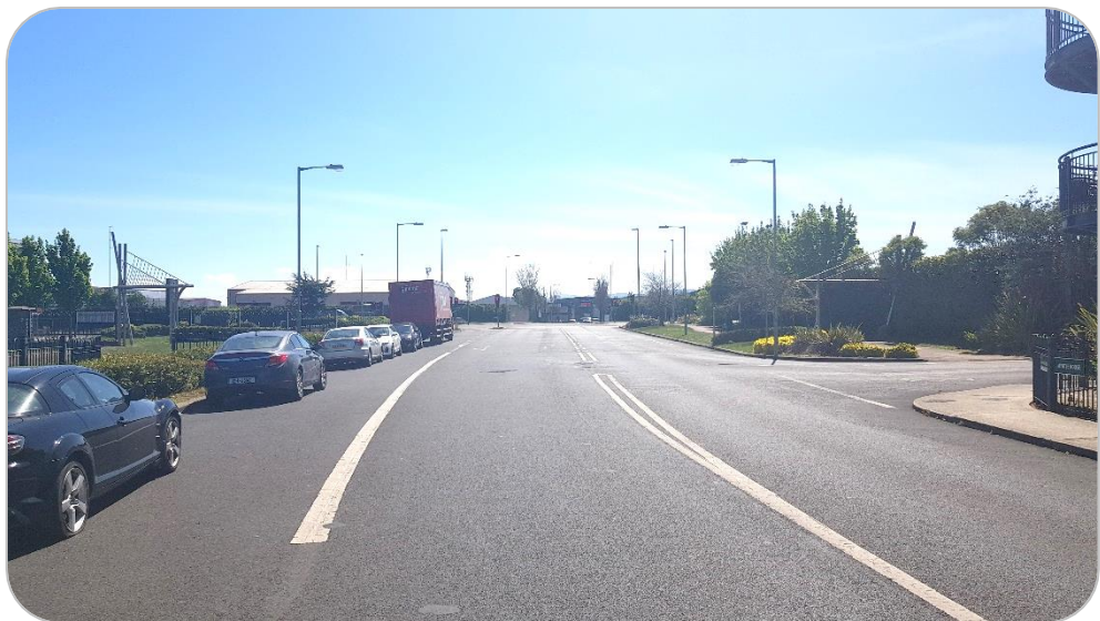
Figure 7 – Longfield Road (view to south to Grange Rd junction)
